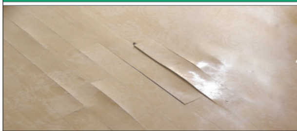
Figure 1. Moisture and pH problems led to strip failure, stressed vinyl composition tile and efflorescence in the seams.
